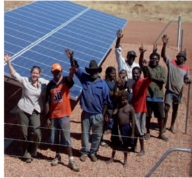
Solar panel installation at a Bushlight community, Northern Territory, Australia.
