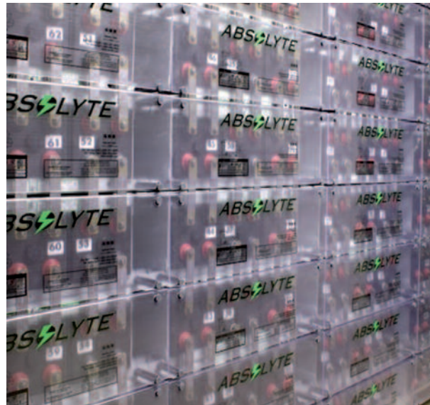
Telecommunication tower in Carol Springs Mountain in Arizona with Absolyte GP.
