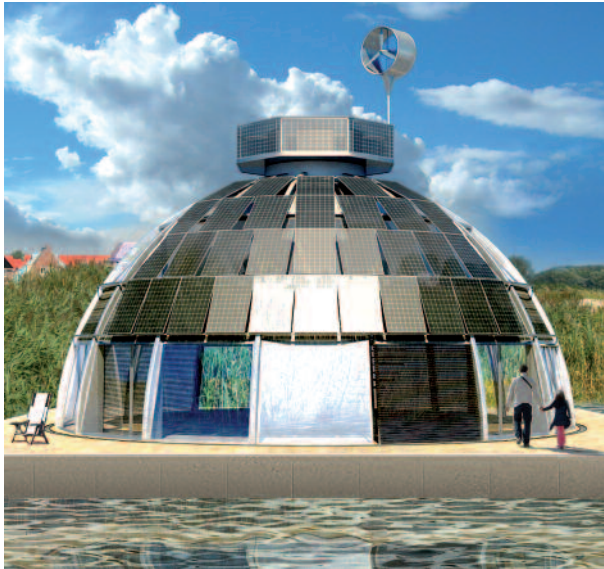
Solar powered igloo in the Netherlands with Sonnenschein SOLAR A600
