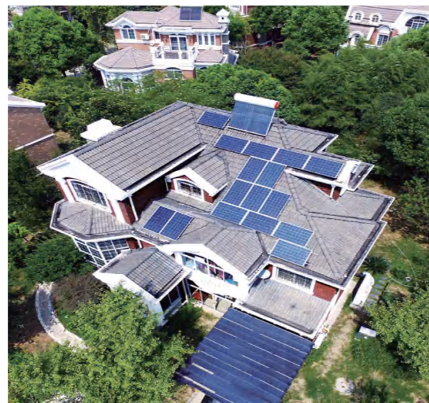
Residential Project in Philippines 3kW
