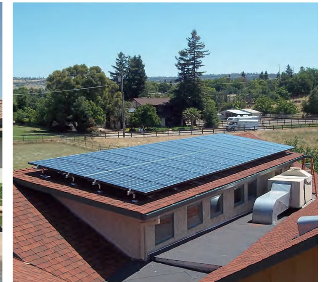
Residential Project in Mexico 5kW
