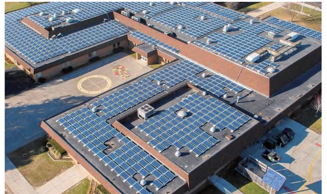
Industrial Project in South Africa 158kW
