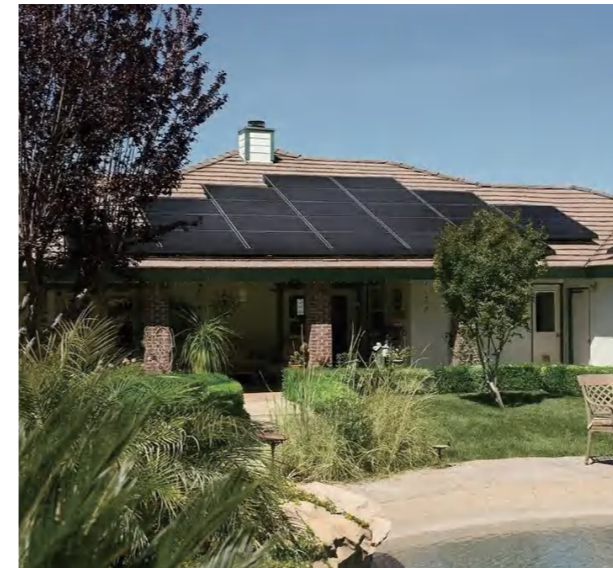
Residential Project in USA 10kW
