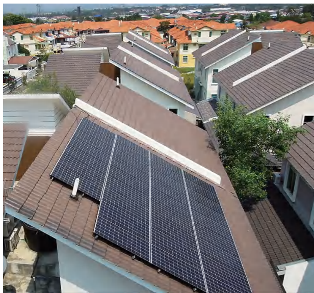
Residential Project in Malaysia 3kW
