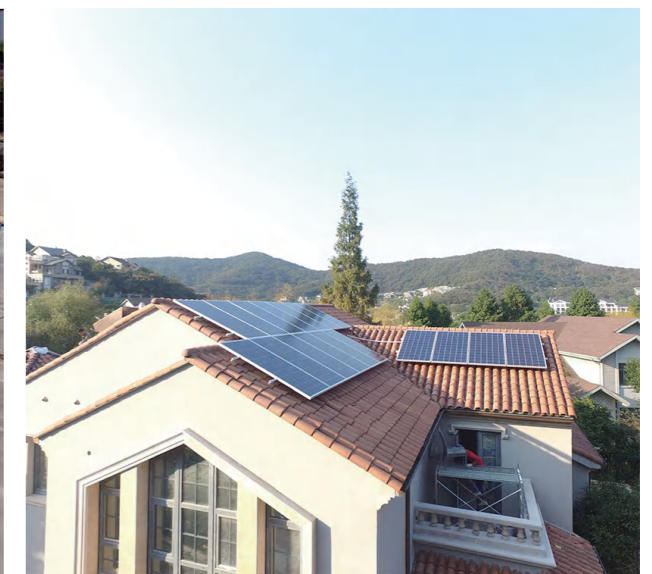
Residential Project in Argentina 5kW
