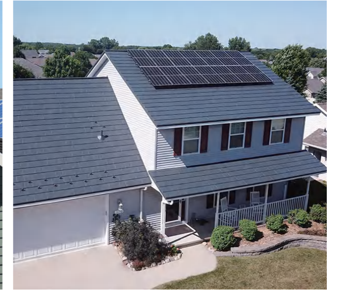
Residential Project in Philippines 3kW
