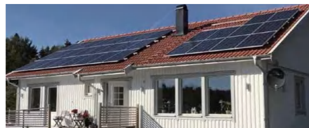
Residential Project in Sweden 10kW
